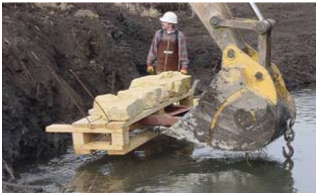
Figure TS140–3 LUNKERS being installed “in the wet”
