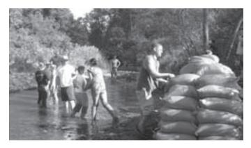
Volunteers filled, hauled, and placed more 900 sand bags in the creek, creating a temporary dam diversion to allow heavy equipment access to build the retaining wall.
